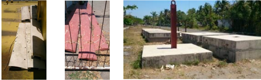
Pictureset 3: Blade farings, arms, 14 mooring blocks, 2 more mooring blocks (sitting next to platform)
